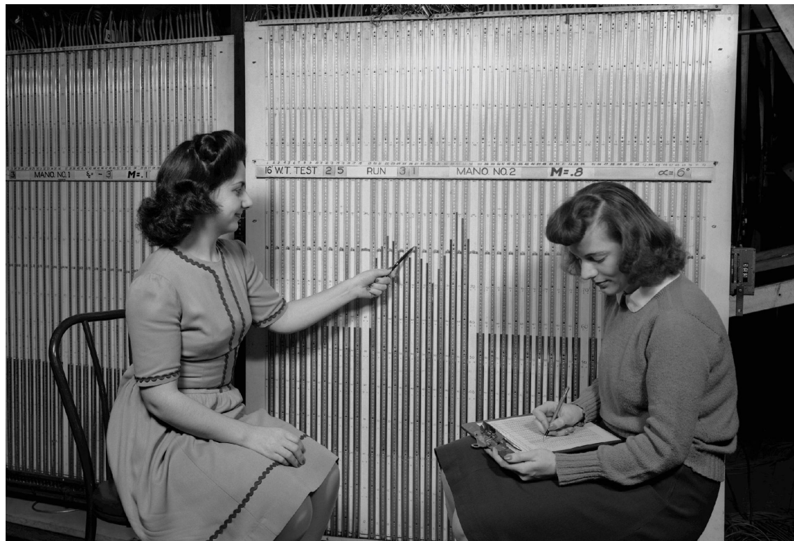
Computers reading the manometer board of the 16-foot wind tunnel, NACA Ames Aeronautical Laboratory, 5 January 1943. NASA, ARC-1943-AAL-4962.
